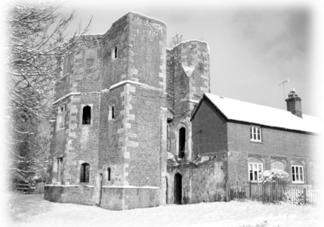
Above: The surviving tower from the south-west, showing the stair tower and the square garderobe (latrine) tower,
